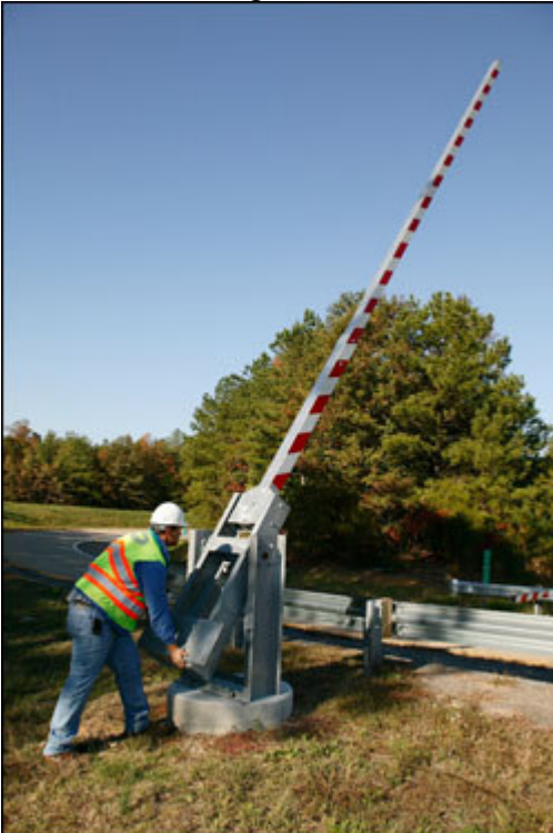
Hurricane gate on I-64
