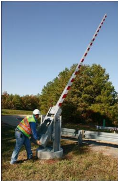
Hurricane gate on I-64
